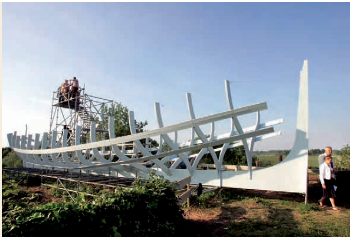
2006 Fort Asperen Ark, a Peter Greenaway Flood Warning
